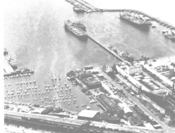
The 51,000-dwt containership S/A Winterberg in Cape Town's Sturrock drydock, with Globe Engineering workshops visible at the left.
