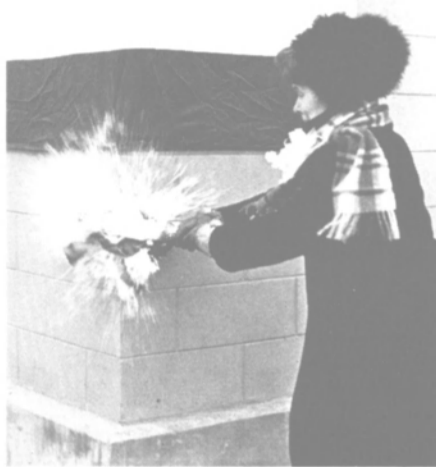
Mrs. Carl A. Brettschneider, wife of the Commandant, Fourth Naval District, christens Sun Ship's new U.S. Navy living accommodations facility.
