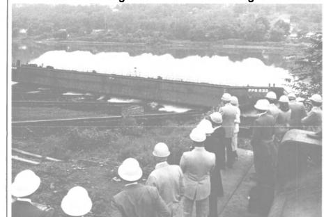
First of 14 new chemical barges for PPG slides down the ways recently at the Hillman Barge and Construction Company yard in Brownsville, Pa.
