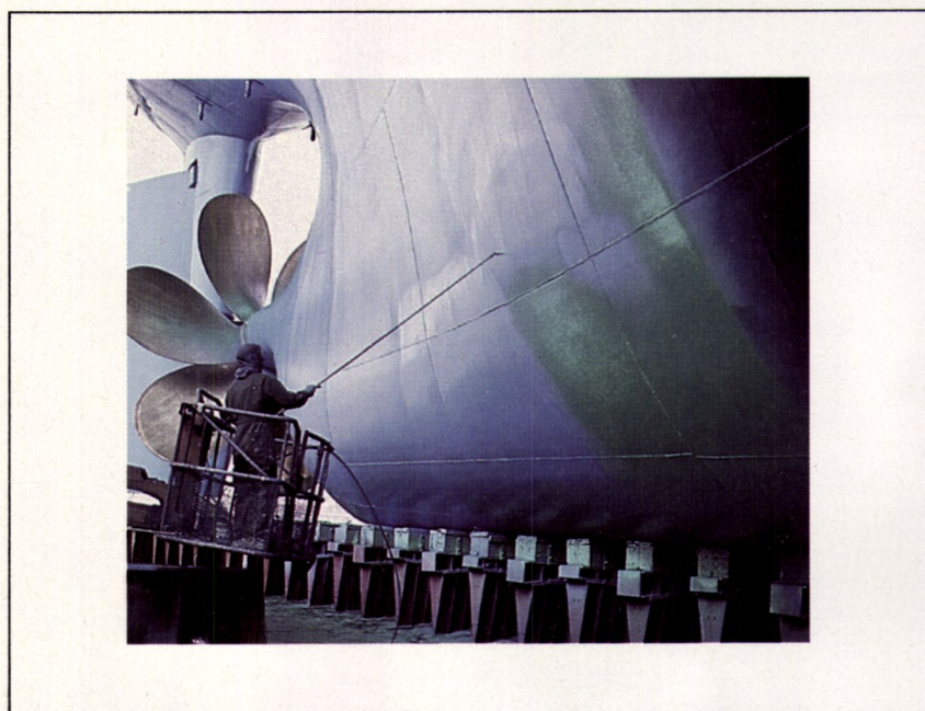
MAUI: dark area – Cathodic Protection Dielectric shield; green – first coat of SPC; blue – second coat of SPC.
