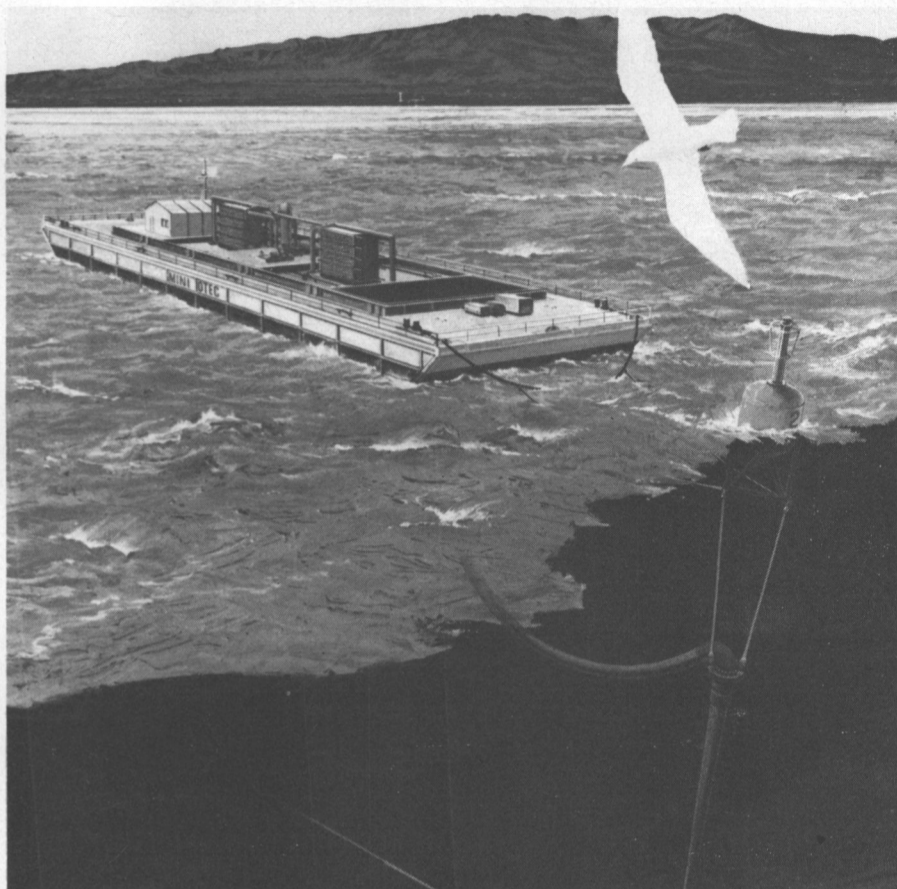
This artist's rendering shows the 50-kw ocean thermal energy conversion (OTEC) plant that the State of Hawaii, Lockheed Missiles & Space Co., and Dillingham Corporation will build and operate, beginning next spring. Fueled by ocean water temperature differences, it will be the first at-sea closed-cycle plant to generate usable amounts of power.
