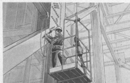
Work basket for one-man steel erection applications.
