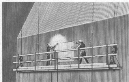
Platform for interior boiler work.
