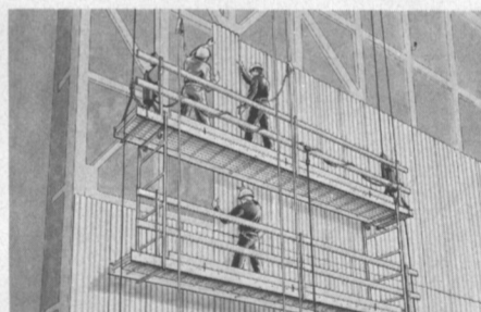
Two-tier platform for installing siding.
