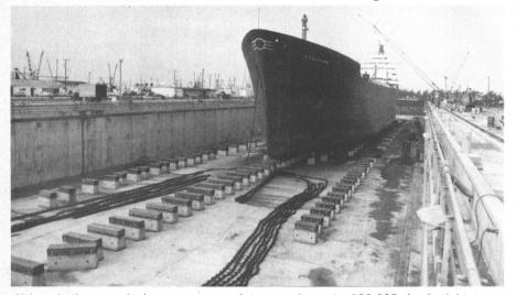
Although the new dock can accommodate vessels up to 100,000 deadweight tons, the Pasadena, a 25,000-dwt tanker, was the first vessel to enter the new 900-foot by 150-foot facility.
