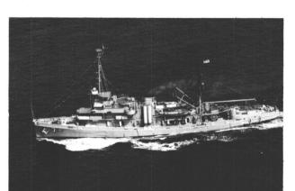
ASR—Submarine Rescue Ship (Fleet Tug) BUILT 1942 251' x 44' x 16' Single Screw-3000 SHP LOCATION: West Coast
