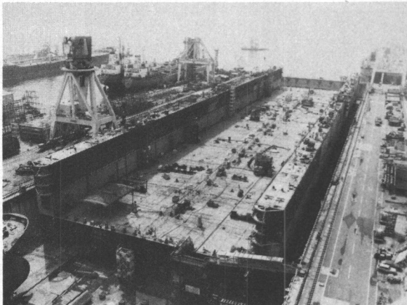
The Port of Portland's new, 982-foot-long floating drydock is shown nearing completion in Kure, Japan.
