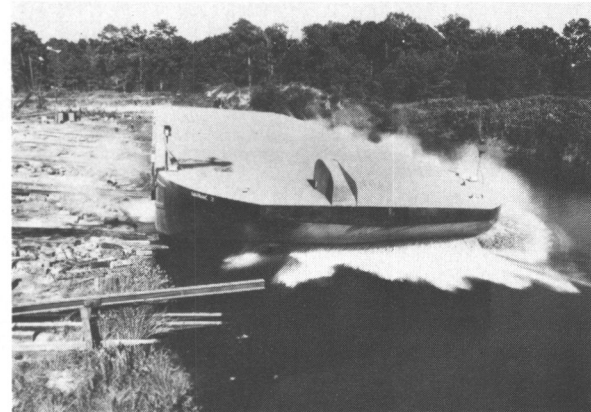
The 240-foot by 72-foot by 16-foot Marmac 3, shown above, is scheduled for operation in offshore oil and gas fields.
