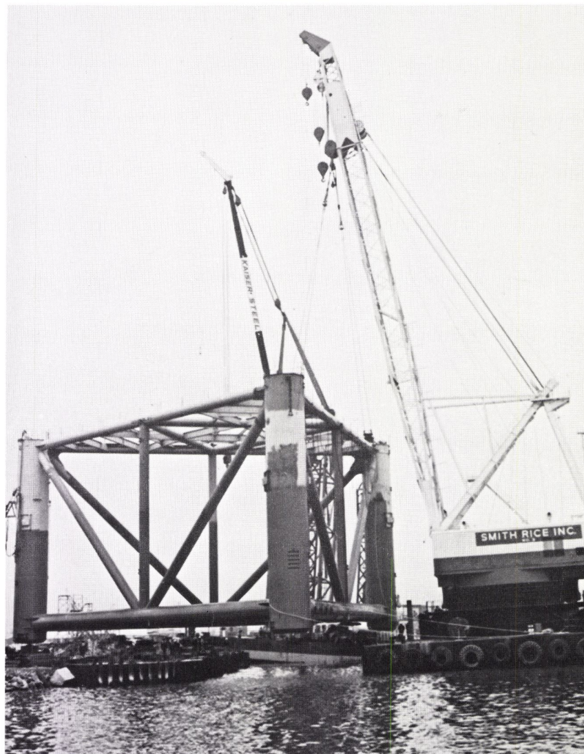
Launching offshore platform, Port of Oakland.
