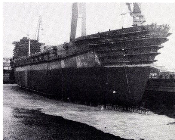
FIRST FLOODING: The Northern Arrow also accounted for another first—she was launched from the first flooding of the Gdynia Yard's new 400,000-dwt-capacity drydock.
