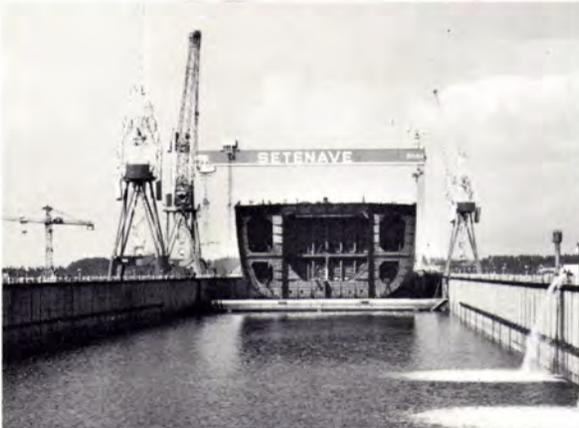
Flooding of the drydock is accomplished by pumps having a total capacity of 400,000 gpm.
