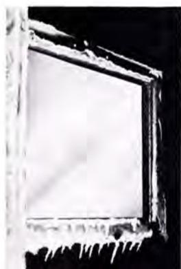
Electrically heated Kearfott window exposed to 45 knot gale, -20° spray.
