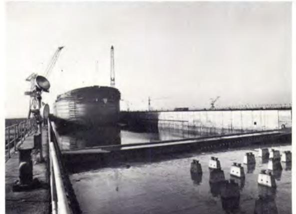
This view shows the hull section after being floated into the drydock and the dock being pumped.
