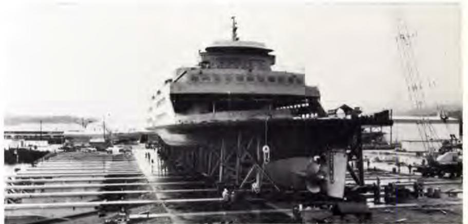
The 3,500-ton ferry, Queen of Alberni, is shown being positioned on launching ways by using the Aero-Caster System, developed by Aero-Go, Inc.
