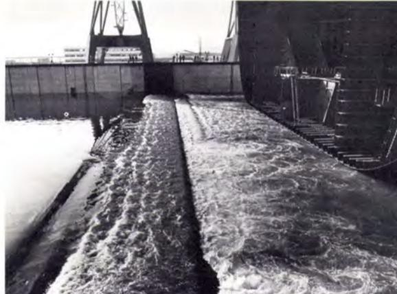
As the repair dock floods, the water flows over the sill into the newbuilding section to float the ship.
