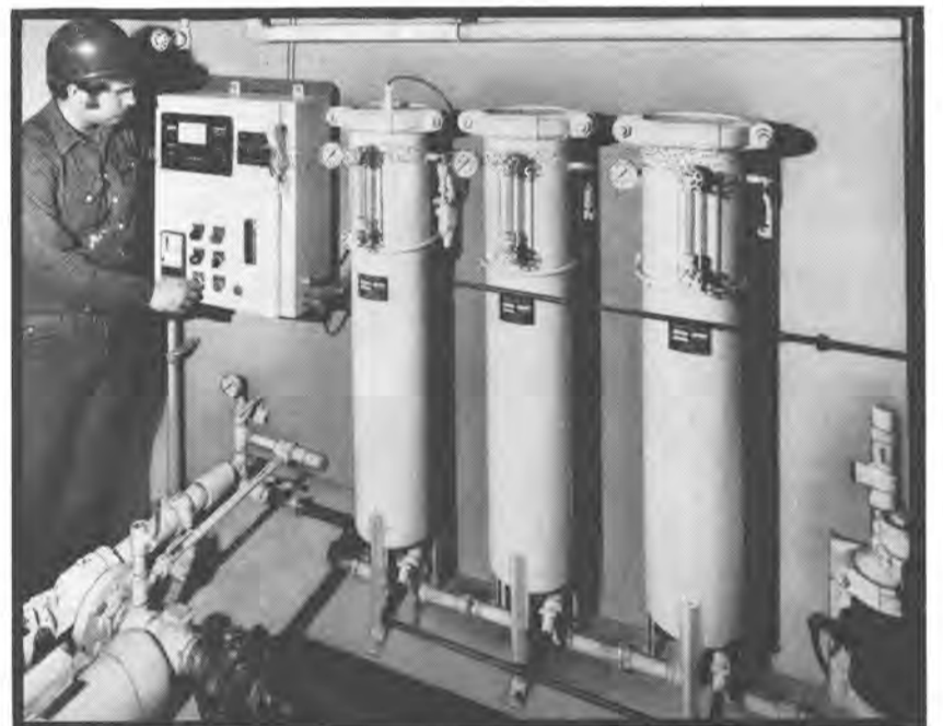
Keene Marine Discharge Control Systems are installed on Federal Barge Line's two largest vessels, the 4-engine, 9000-hp, 184-foot M.V. America and its sister ship M.V. United States (shown here).
