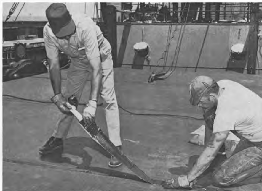
Strips are quickly positioned over the joint area to be sealed. Strips are butted end-to-end, providing a watertight seal the length of the joint. Foot pressure forces the instant-bonding plastic into intimate contact, bridging the joint with a flexible, watertight seal.
