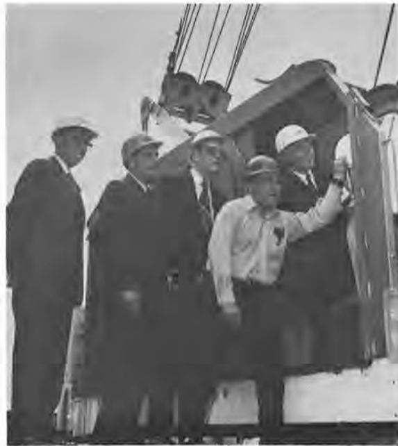
Robert Dickey III (sitting at the controls), president of Dravo Corporation, headed the team that broke ground as full-scale work began on the $5-million expansion of the company's Neville Island Plant.
