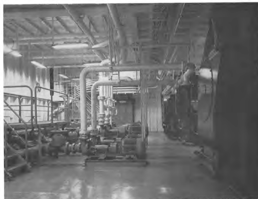
View of the mud pump room showing the triplex mud pumps on the right, the centrifugal supercharging pumps in the middle and the mud suction manifold on the left. The mud pits are located beyond the bulkhead seen at the extreme left.
