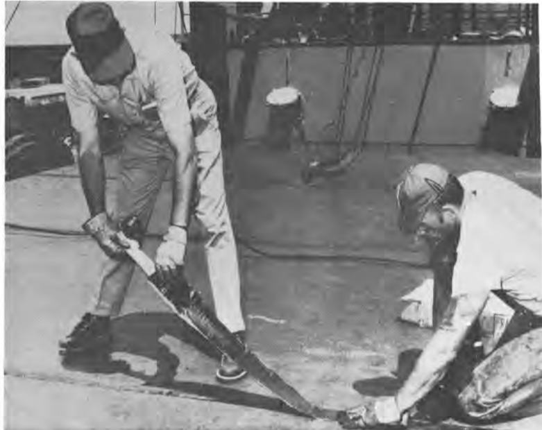
Strips are quickly positioned over the joint to be sealed. The self-sealing material is placed end-to-end to provide a watertight seal the length of the joint.
