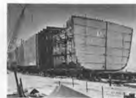
Catug construction seen from bow portion
