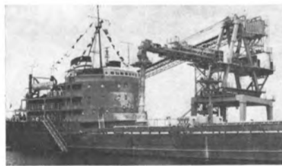
Bulk Loaders —This bulk loader, operated by one man, handles 750 Long Tons per hour of Alumina; 1000 Long Tons per hour of Bauxite. Designed with slewing upper tower and hinged apron.
