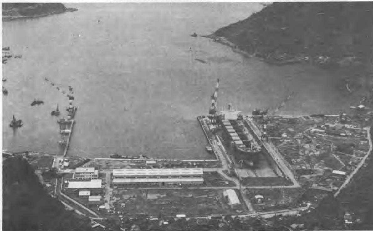
Aerial view of the new ship-repair yard at Yura, Japan. This new facility with its first repair job in the large drydock was built to fill a need for servicing large tankers and container ships having deep drafts.
