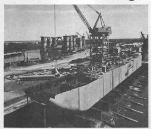
The starboard hull for the Zapata Ugland is shown above on the Beaumont yard building ways. In the left center, foreground, is the semisubmersible Pacesetter I, built for Western Company of North America. Beyond the Pacesetter I is the Zephyr I, a semisubmersible under con-
