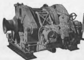
2—ALMON A. JOHNSON Stern Anchor Winches as removed from L.S.T. Vessels, line pull rating 100,000 pounds at 10 FPM in low gear, complete with Contractor Panels, Resistors, and Master Switches.
