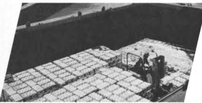
Fork lift discharges LASH barge load of beer in palletized Shrink-Paks.
