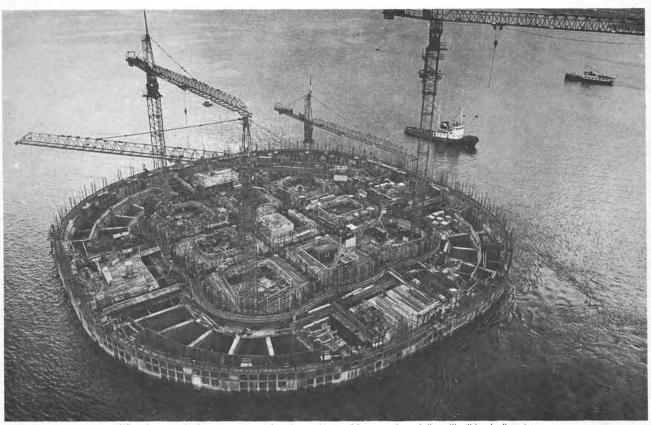
When the one-and-only-one sea voyage takes place under tow of four tugs, the tank "vessel" will break all maritime records for weight moved, draft below the waterline, beam of vessel and sheer volume of a man-made object in controlled sailing. The photo above shows the tank just prior to being anchored in Hillevagen Bay at Stavanger.
