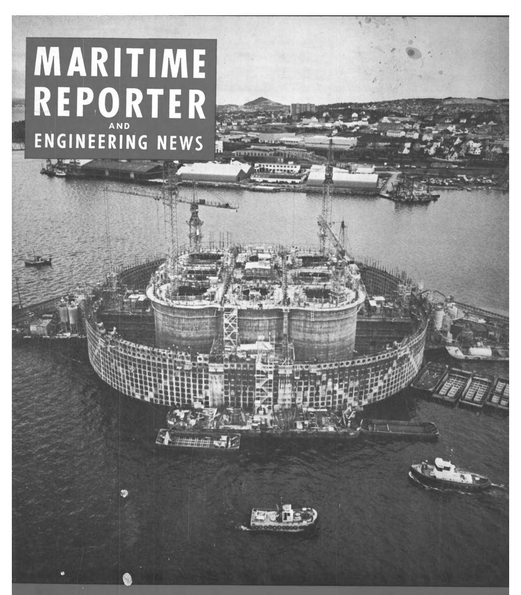
World's Largest Ocean "Vessel" Will Be Towed 250 Miles Out Into The North Sea To Function As One-Million-Barrel Oil Storage Tank
