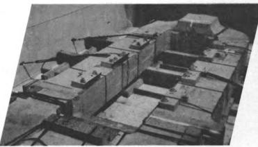
Electrical machinery heavy lift (142 L.T.) is secured in LASH barge for export.
