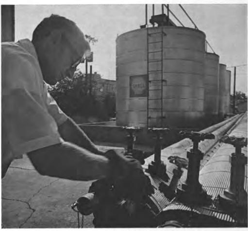
E. J. Wheeler, Manager of Marine Oil Services, Inc., opens an outlet valve so that ALEXIA Oil can be pumped at 55 gals./minute into a waiting tank boat. Four insulated 10,000 gallon storage tanks hold Shell lubricants at a constant 120°F., permitting fast flow in any season.
