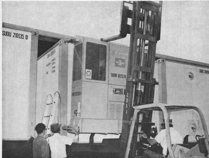
69NK simply clips to the container for shore duty, using the same air connections as aboard ship.
