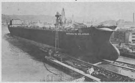
The Marques de Bolarque shown on the ways at the Sestao yard, built with both a bulbous bow and stern, has a relatively narrow beam for transiting the Panama Canal.
