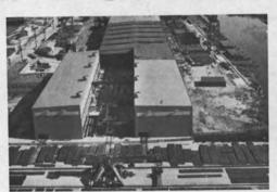
Fabricating shop was lengthened by nearly 600 ft and a roll shop added. Plate handling has been improved by the new electric hammerhead crane (foreground and above) and by electric transfer cars which bring stock from the storage yard into the shop.
