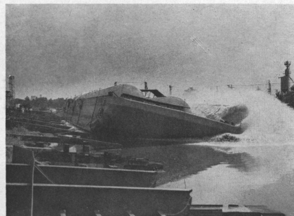
FIRST OF FIVE: The inland service LPG pressure tank barge Cherokee slides down the ways of Bethlehem Steel's Beaumont, Texas, shipyard. She is the first of five similar barges being built by Bethlehem for Warren Petroleum Corporation. Designed by Bethlehem for the transportation of butane, she has an overall length of 175 feet, beam of 42 feet, depth of 12 feet and loaded draft of 8½ feet at her 10,000-barrel capacity. She is equipped with two cylindrical pressure tanks, 16 feet 9 inches internal diameter, by 141 feet internal length, with hemispherical heads. She will be fitted with rain shields in the openings between the tanks, and between the tanks and tank hold compartments. Built under U.S. Coast Guard inspection, the vessel is classed with the highest rating for craft of her type by the American Bureau of Shipping.
