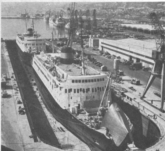
GROIGNARD CONVERSIONS: Groignard Shipyards of Marseilles, France, recently completed the conversion of two Danish car-ferries into cruise ships. The vessels, Dana Corona and Dana Sirena, each 408-feet 6-inches long, were delivered to their owners, Det Forende Company of Copenhagen, Denmark, on schedule. Shown above are both vessels being completed simultaneously by the Groignard Shipyards in Drydock No. 9 of Marseilles, with the bow of one vessel in the raised position to permit the operation.
