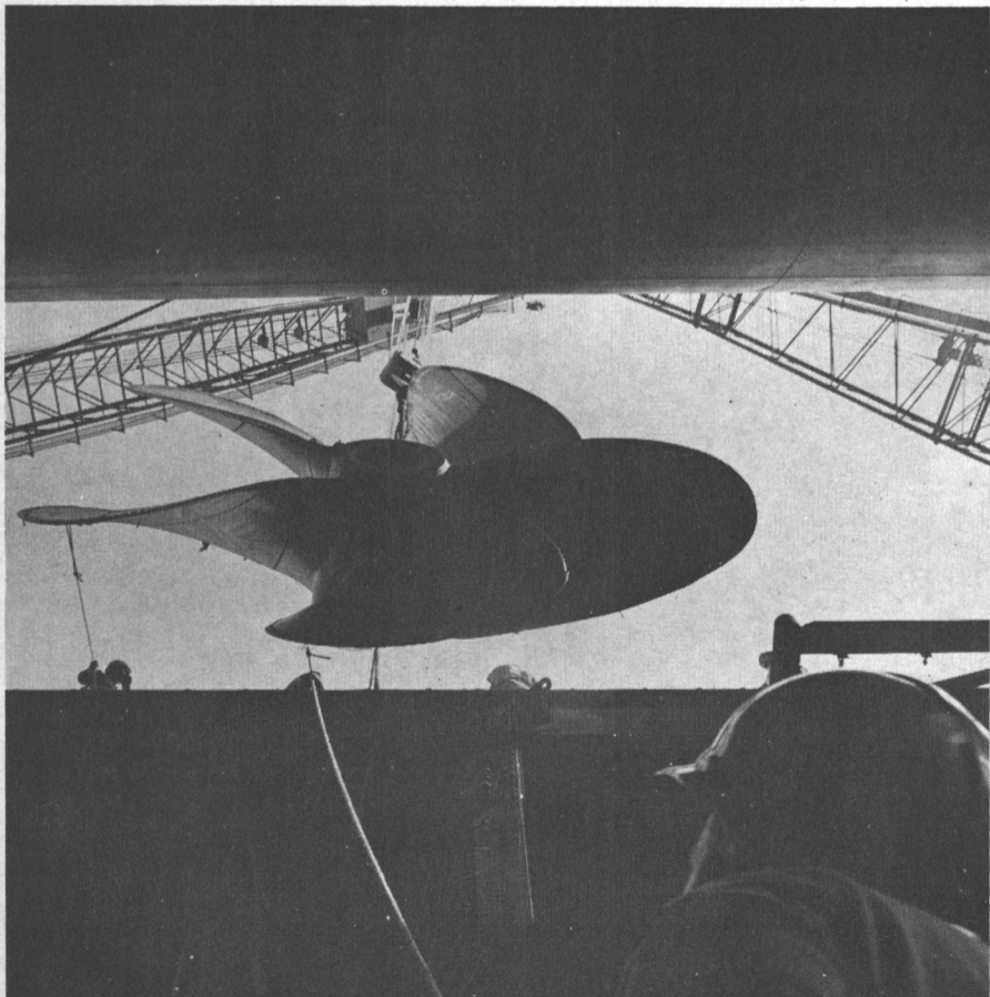
The 45-ton Ferguson propeller being lowered sideways between the building-basin wall and the ship's cantilever stern, since normal access was obstructed by work on the 2,000-ton capacity elevator platform. The propeller has a diameter of 23 feet.
