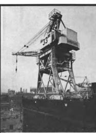
Each wingwall carries a 60-ton crane with 90-ft boom. Centerline lift with spreader bar: 120 tons.
