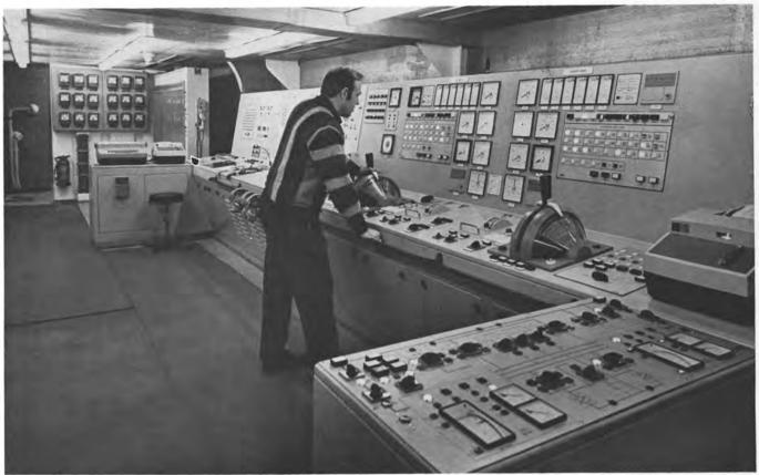
The air-conditioned engine control room contains all the controls and alarms for the main and auxiliary machinery.
