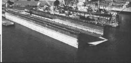
New dock can lift 65,000 tons and accept a vessel of max 150-ft beam and 31-ft draft. Pontoon is 20 ft deep, has 800-ft-long unobstructed deck—plus two 50-ft, grate-type aprons. Its 2,000 pumping hp can lower and raise the unloaded dock in less than 40 minutes.
