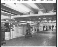
Spacious safety decks at the 68-ft level in both wingwalls house the pumps, motors, substations, and other equipment. They are compartmented by watertight bulkheads.
