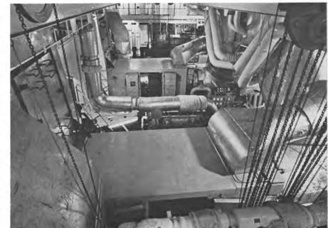
View of the engine room shows the two gas-turbine units with the doors to the soundproof engine enclosures open. The tops are removable for easy and fast maintenance.
