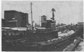
STEEL SELFPROPELLED LIGHTER 100' x 30' x 7' Draft M.E.—GM 12-567A Aux. Gen. G.M. 2-71 Hoist Eng. G.M. 2-71
