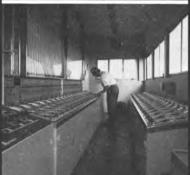
Control of pumps and flooding for all 40 ballast compartments through banks of buttons and indicators is centered here in the control house atop the west wingwall.
