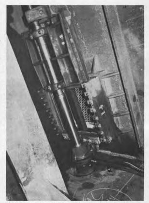
SIGMA type port valve in bulkhead provides for the intertank free-flow system and greatly reduces cargo piping.
