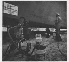
A barge in Harvey, La., being coated with 98 percent solids glass-filled polyester resins using a Spee-Flo Commander Special model.
