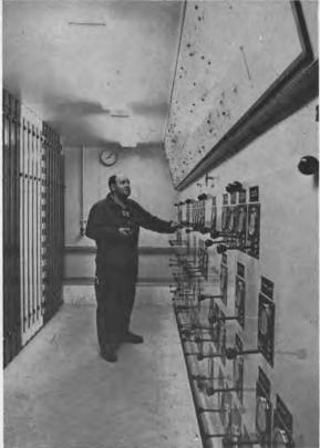
Cargo control room from which most cargo valves are remotely operated has mimic diagram of the cargo system.
