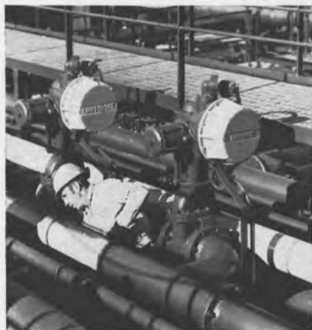
New Limitorque XPM valve operators control cargo flow.
