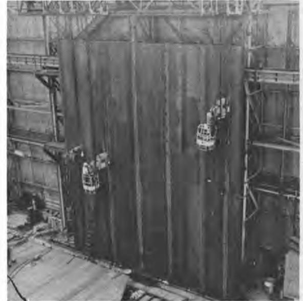
Joining panels by use of the electro-gas welding process.
