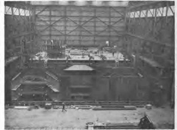
Vertical module construction. This unique method facilitates positioning of subassemblies and permits concentration of labor and tools in a small area.
