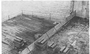
Temporary steel reinforced 4-foot bulkheads were erected and sealed prior to damaged vessel's arrival to prevent leakage from each end of drydock at Todd New Orleans.
