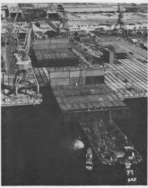
Massive launch pontoon sections move forward on rails from the construction site to the launching barge in the Pascagoula channel.
