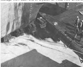
Entrapped oil from the vessel's tanks and oil water is chemically treated as it is pumped from the barricaded drydock to the disposal barge.
