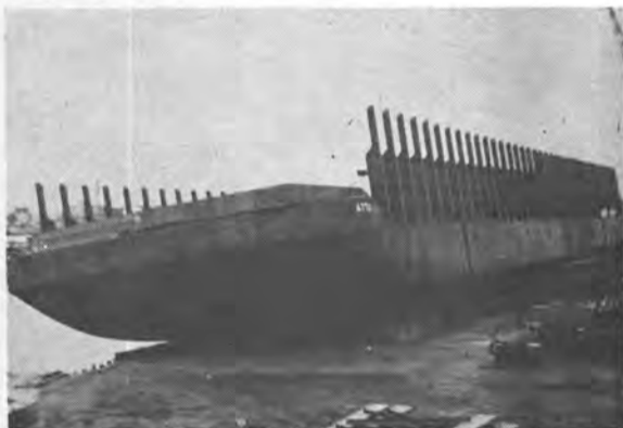
TODD DELIVERS 400-FOOT ALASKA-BOUND RAIL-CAR BARGE: The barge Attu shown on the ways before launching at Todd Shipyards Corporation (Houston Division) was recently delivered to Harbor Tug & Barge Company of San Francisco. The Attu is the first of two rail car barges measuring 400 feet by 99 feet 6 inches by 20 feet to be built by Todd-Houston for Harbor Tug & Barge. These are the largest deck cargo barges ever built in the Houston area. The unmanned, non-self-propelled barges are designed to carry 64 rail cars per trip and will be classed *A-1 for Pacific Ocean service. The Attu was specially equipped with 74 thirty-foot-high stanchions which will allow the vessel to transport approximately 12,000 tons of 48-inch diameter pipe to the Prudhoe Bay area for the first portion of the 800-mile oil pipeline to run from Prudhoe Bay to Fairbanks and across to Valdez on the upper rim of the Gulf of Alaska. After the maiden voyage of the Attu, the stanchions will be removed and the rails will be installed on the deck for the vessel's second trip as a hydro-train. Delivery of the second barge Adak at Todd-Houston is scheduled for next month.
