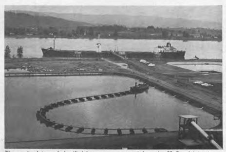
Thousands of tons of slurrified iron ore are pumped from the SS Oread into storage pond at Oregon Steel Mills. Slurried ore is reclaimed by the dredge on the pond.
