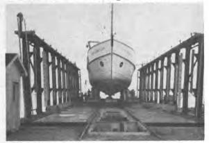
The trawler Jean Cabot was the first vessel to be drydocked and transferred for winter storage on the new railway dry dock and transfer system at Caraquet.
