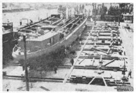
300 ton side transfer system used for barge construction with launching by means of side-haul railway, Dordrecht,
