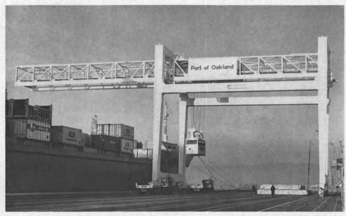
Built by PACECO for the Port of Oakland, this Low Profile Portainer not only loads and unloads container ships but also services the storage
