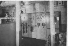
Electrical switchboard contains distribution panel (!eft), generator panel (center), and capstan control (right).
