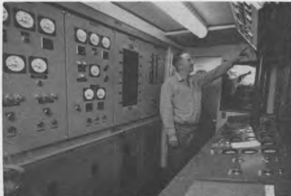
Engine controls and gauges are centralized in a sound-proofed room at the forward end of the machinery space.
