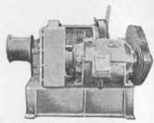
American Hoist and Derrick Company Winches with Westinghouse Motors. 50 HP, 230 Volts DC. complete with Contactor Panels, Master Switches, and Resistors.
