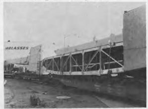
In Wisconsin-Marinette built the all-aluminum craft, complete, and then removed the large bow ramp and sawed the vessel in half lengthwise. The entire craft was then loaded on three flatcars and shipped to Tatco Shipbuilding in San Diego, Calif.
