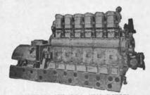
ENTERPRISE 250 KW DIESEL GENERATOR SET 450 HP Enterprise DSG-6 diesel engine—4 cycle 6 cylinder; with air starting; direct-connected to G.E. 250 KW 3-wire compound wound 120/240 DC generator. 450 RPM—ex C1-MAV-1. 206" long—60" wide—105" high—47,000 lbs ELLIOTT 250 KW DIESEL GENERATORS
