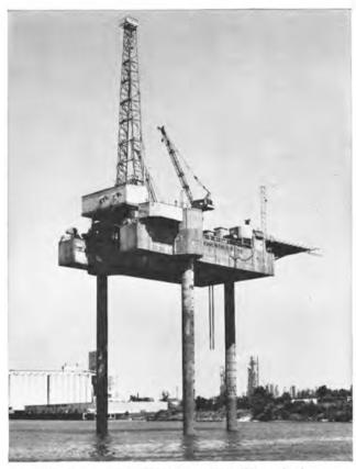
This self-contained mobile oil-drilling platform, shown in elevated position during jacking trials, operates in water depths to 125 ft. Our Beaumont Yard has built such rigs capable of operating year-round in water depths to 250 ft.
