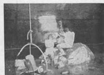
Damaged Liberty hull was sealed with CORDOBOND resins and fibre glass prior to refloating-Costly gas freeing was eliminated.
