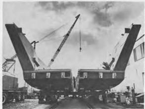
At San Diego-When the two sections of the landing craft are aligned, they are welded together by pairs of welders, starting at the craft's center and progressing at the same rate in opposite directions. New shielded aluminum arc-welding equipment insures excellent penetration at rapid welding rates.
