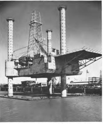
This sister rig to that on the left shows the drilling platform elevated 42 ft above the huge foundation mat. The mat imparts excellent stability to these rigs in a wide range of bottom conditions.
