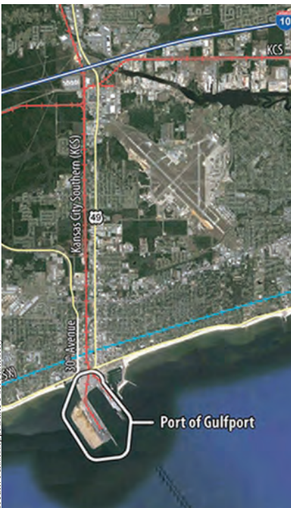
Aerial photo of Port of Gulfport after Hurricane Katrina.
