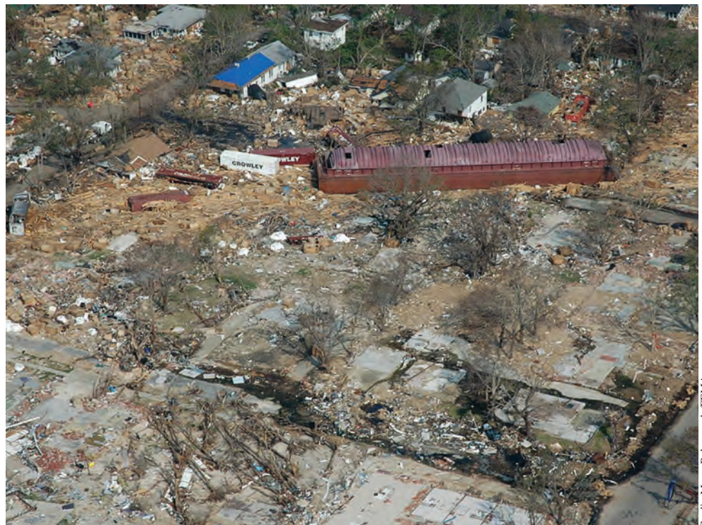
The results of the 25 foot storm surge, buildings destroyed and containers scattered, at the Port of Gulfport following Hurricane Katrina.
