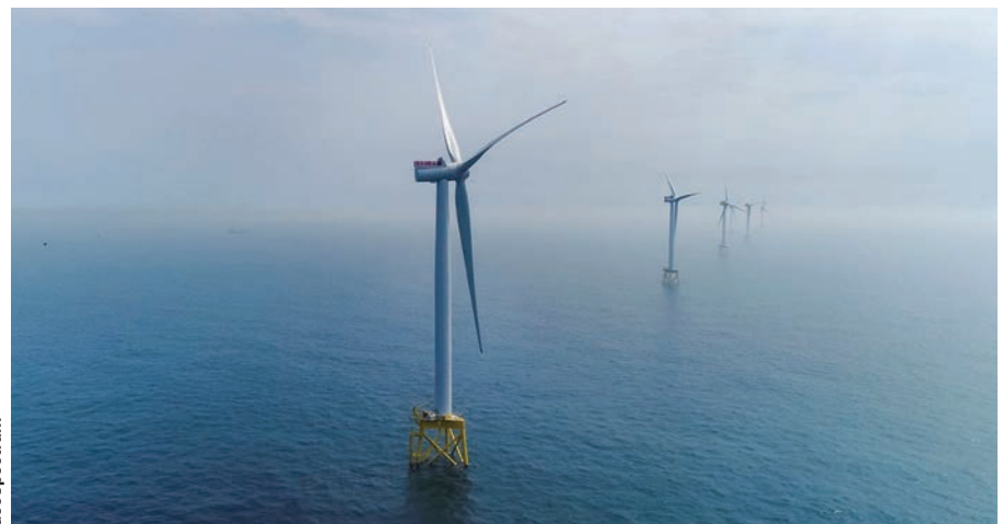
CWind Taps Rovco for Offshore Wind
