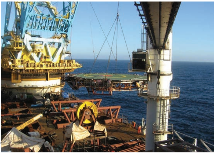
Lifting the heli-deck off the Miller platform.
