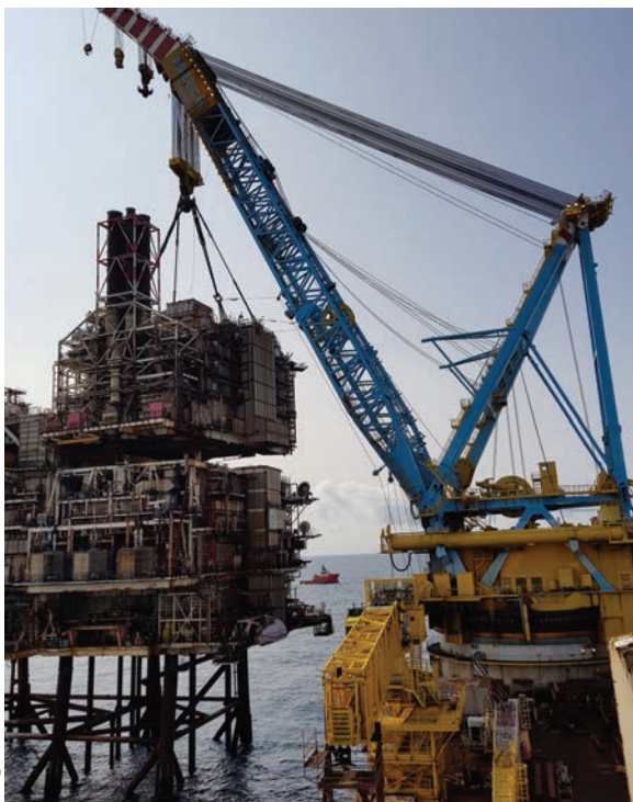
Left: Saipem's S7000 lifting the accommodation module from BP's Miller platform.
