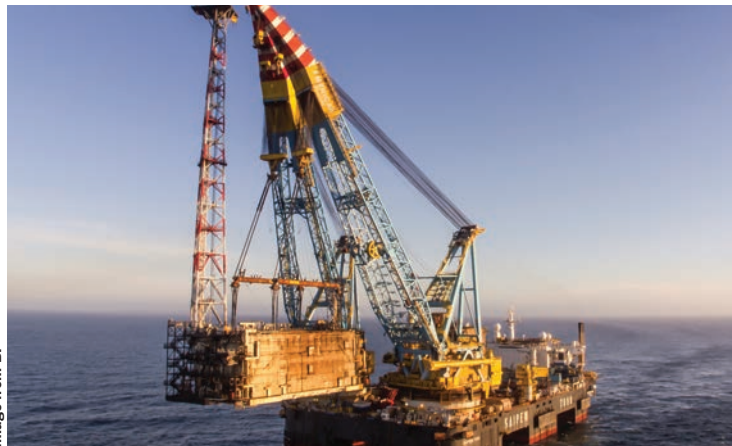
Right: The derrick being lifted off the Miller platform.
