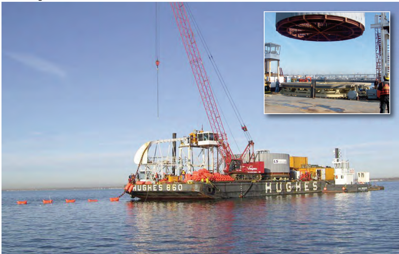
Cable being installed from turntable.
