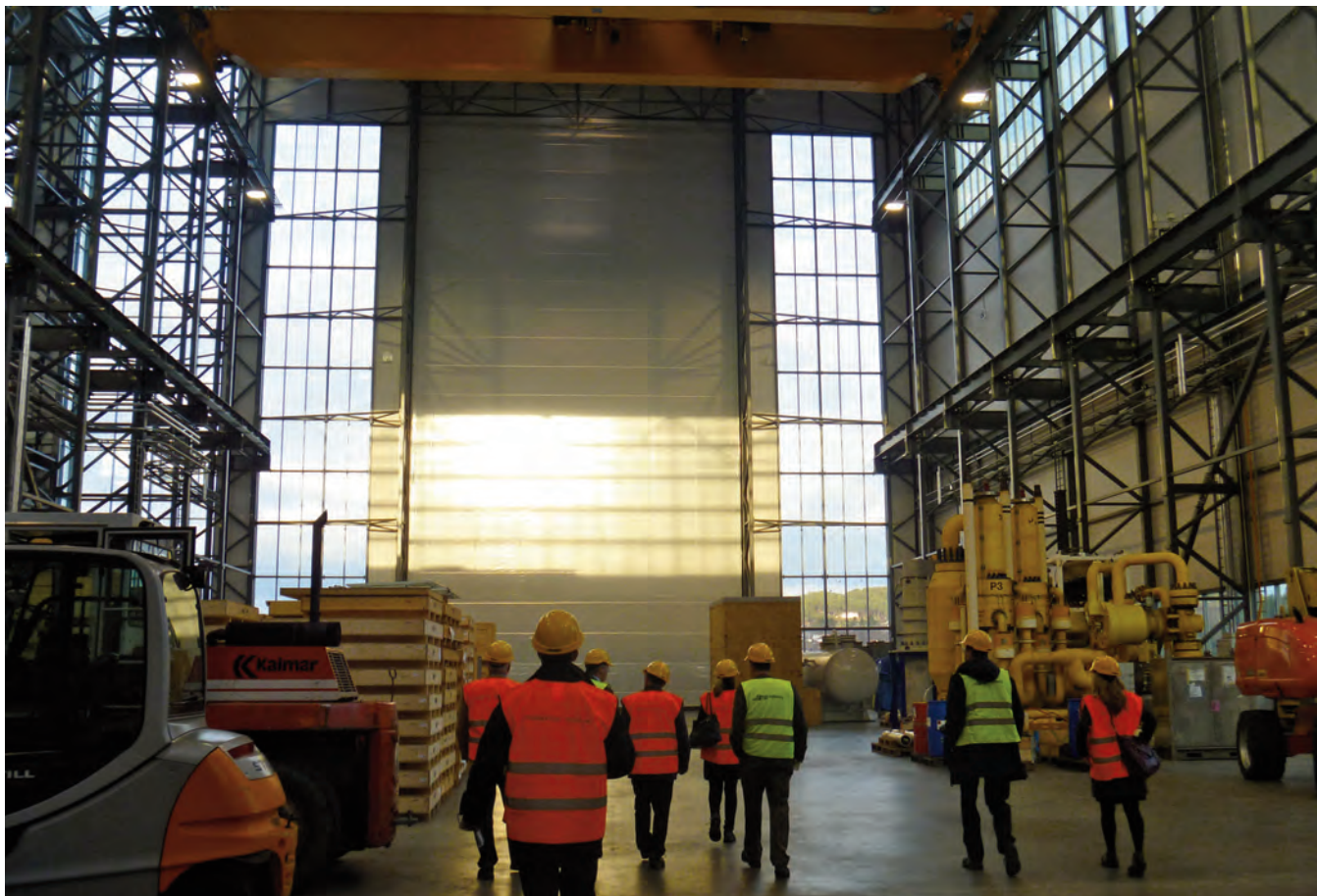
Inside Framo Engineering's large new facility at Horsøy, near Bergen, Norway.
