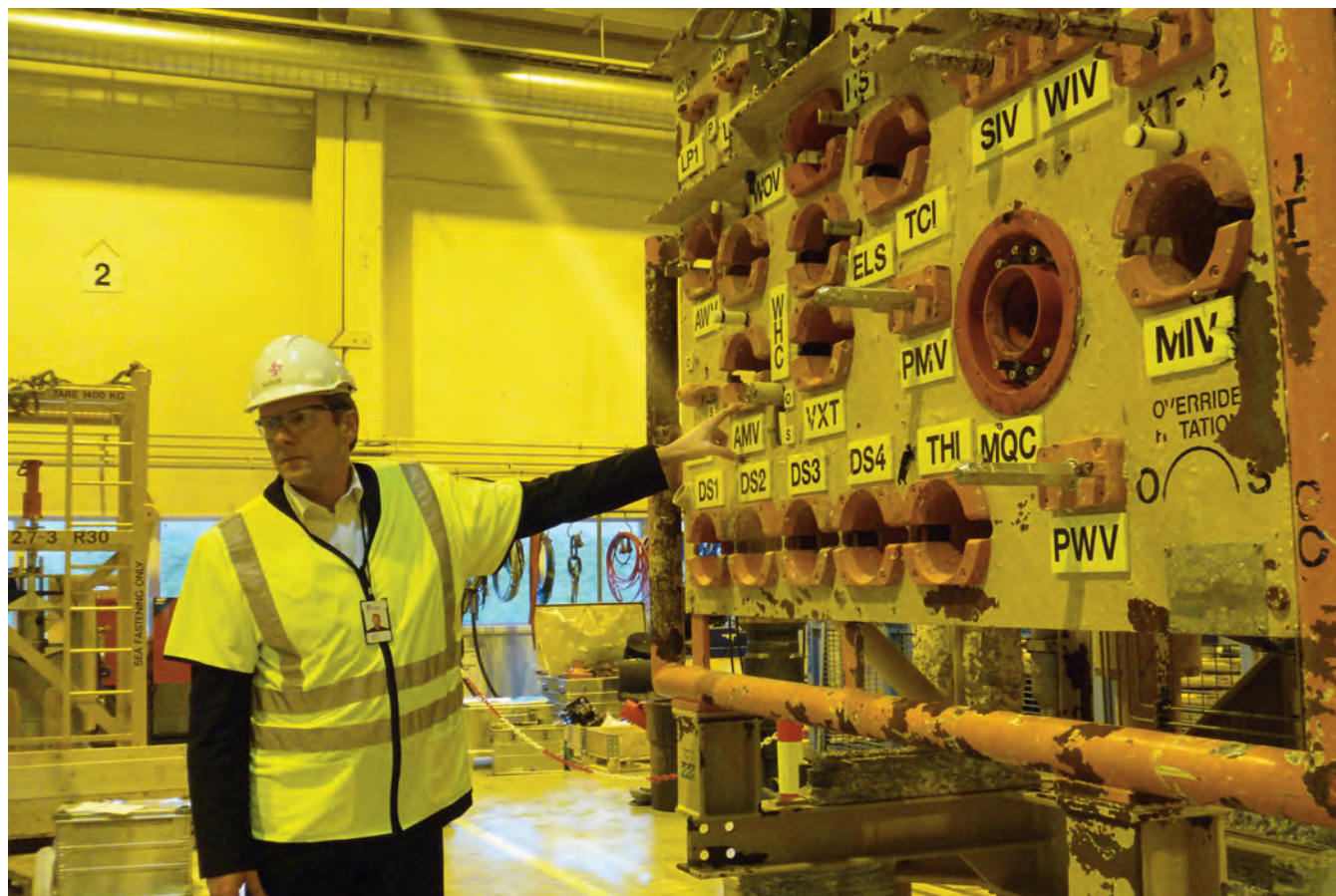
Ove M. Kallestad, Vice President Subsea Technology and Operations at Statoil, showing Marine Technology Reporter a subsea christmas tree at Statoil's Subsea Pool at Ågotnes, near Bergen, Norway. November 2011.
