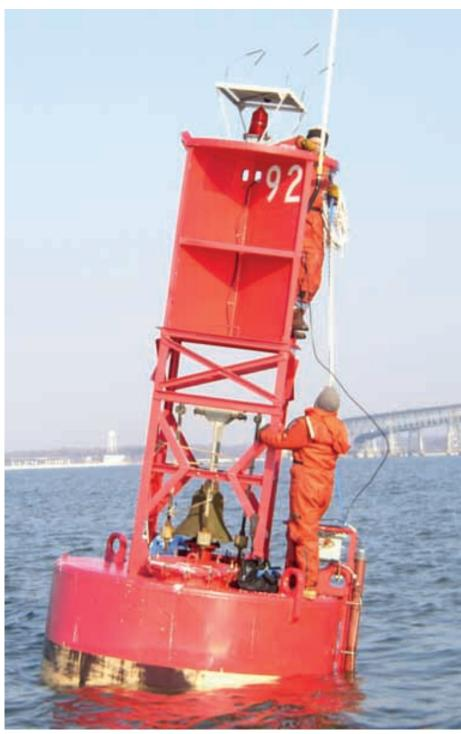
NOAA Ports Technicians at work installing a buoy-mounted current monitoring system in Chesapeake Bay.
