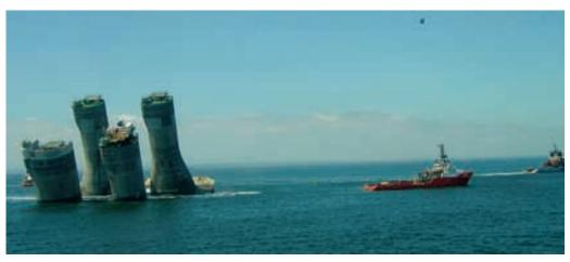
Above: The tow out of concrete gravity base substructures (CGBS) for the Lunskoye A (LUN-A) and Piltun-Astokhskoye B (PA-B) platforms.
