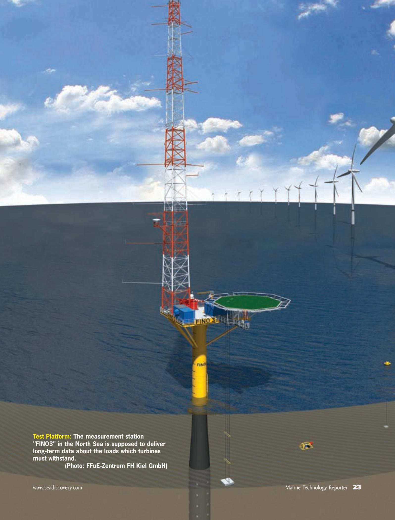
**Test Platform:** The measurement station "FINO3" in the North Sea is supposed to deliver long-term data about the loads which turbines must withstand.
