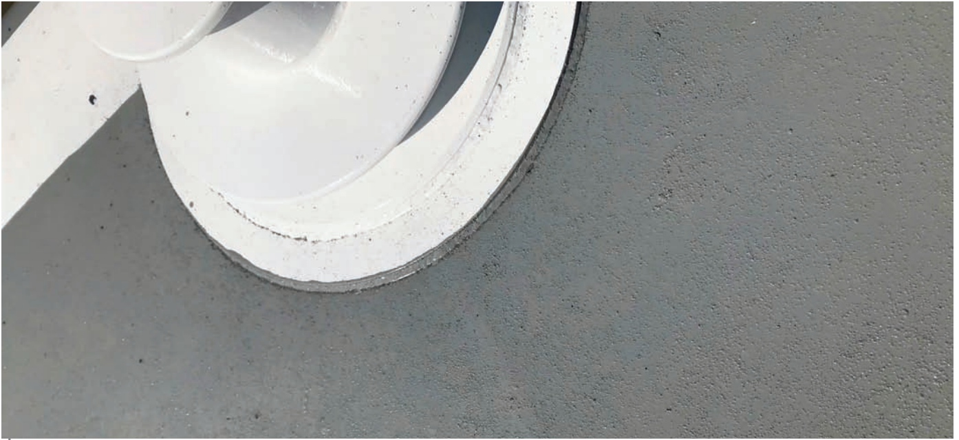
The topside deck and other walkable surfaces of the new barges feature a non-skid aluminum oxide coating system to enhance operator safety.
