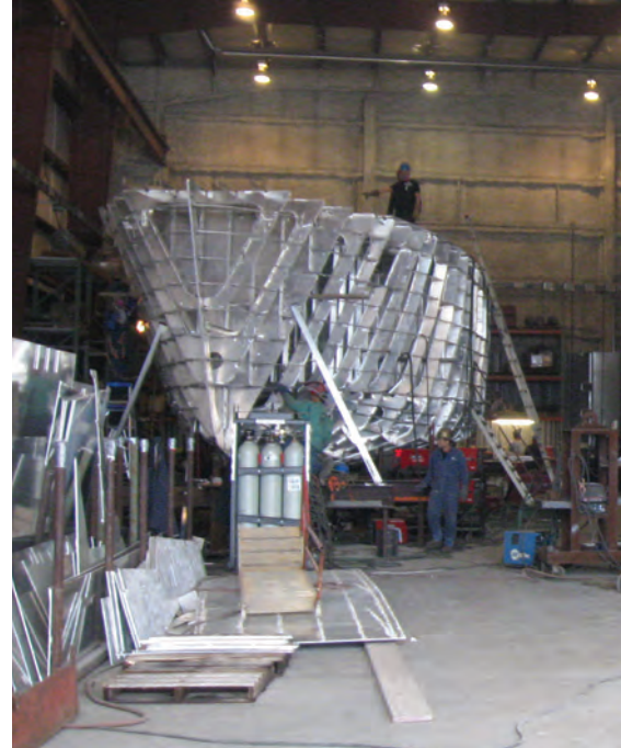
Construction underway at the Great Lakes Shipyard.
