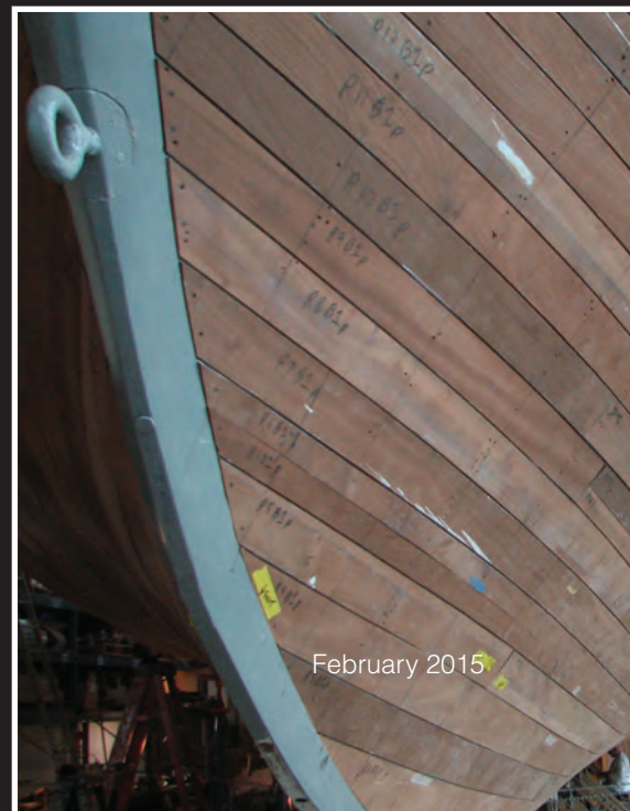
First layer of planking fastened to boat
