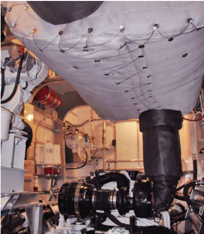
Above & Below: Installing and retro-fitting an exhaust particulate filter system can create many space constraint challenges.
