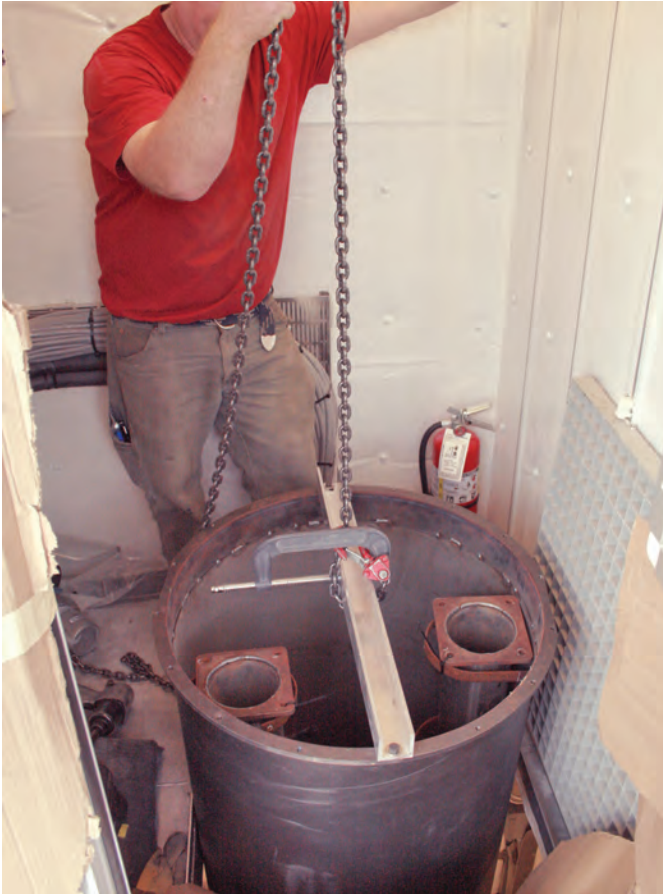
Above & Below: Installing and retro-fitting an exhaust particulate filter system can create many space constraint challenges.
