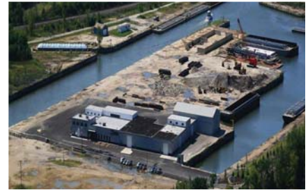
ACL expands warehouse space
