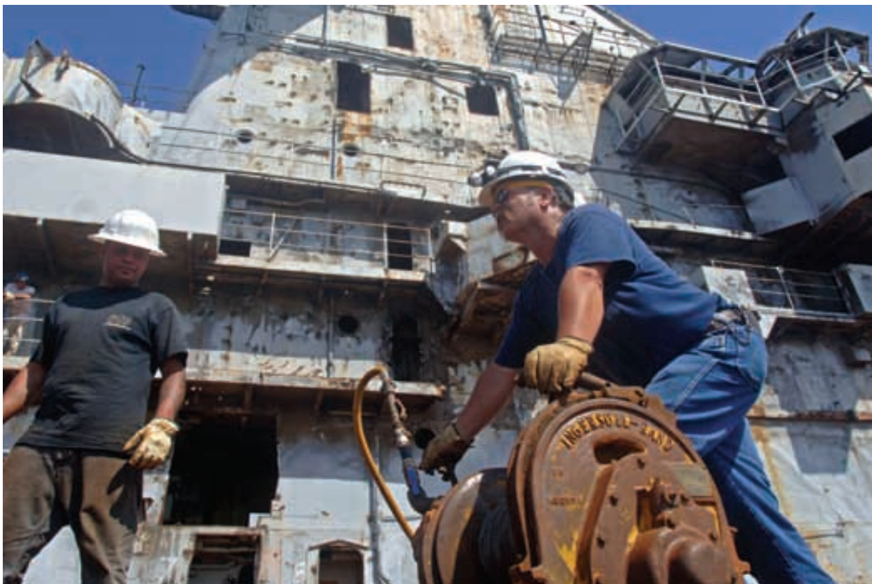
Resolve Marine Group employees, left, Aaron Nahapetian and Robert Lee Jr., begin pulling cable in off the flight deck aboard the decommissioned aircraft carrier USS Oriskany (CVA 34) in preparation for the ship's scheduled sinking. Oriskany is scheduled to be scuttled 22 miles south of Pensacola in approximately 212 ft. of water in the Gulf of Mexico May 17, 2006, where it became the largest ship ever intentionally sunk as an artificial reef. After the Oriskany reaches the bottom, ownership of the vessel will transfer from the Navy to the State of Florida. U.S. Navy photo by Journalist First Class Jackey Bratt
