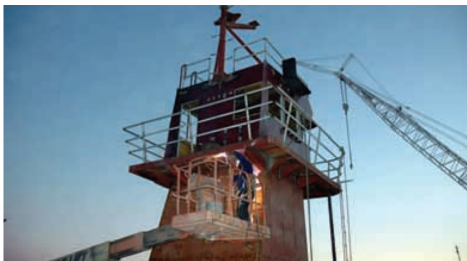
Often the building of double-hulled barges, leads to repair/rework of the tugs designed to push the barges. In this photo, a raised pilothouse for a tug is constructed at Bollinger Marine Fabricators for an undisclosed customer.
