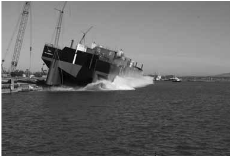
The first of six barge hulls for ATBs being built by VT Halter Marine for Crowley Maritime Services is launched in late December at Halter's Pascagoula shipyard.
