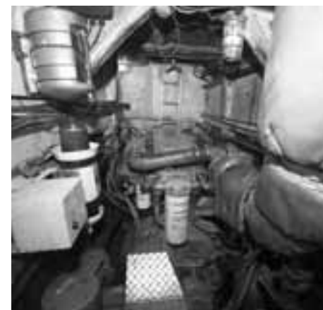
One of each boat's two Detroit Diesel Series 60s, this one in the starboard hull. Under full service conditions, the low-emission engines are said to get by on about 20 gallons per hour. (Photo: Don Sutherland.)
